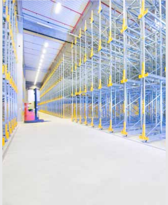
A view of the 42,000 m 2 compact warehouse
